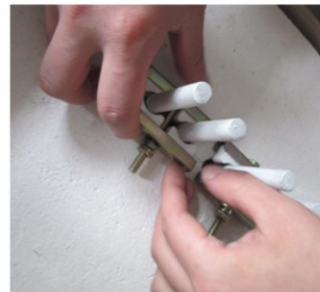
Step 8: Tighten up the Porcelain Clamp
